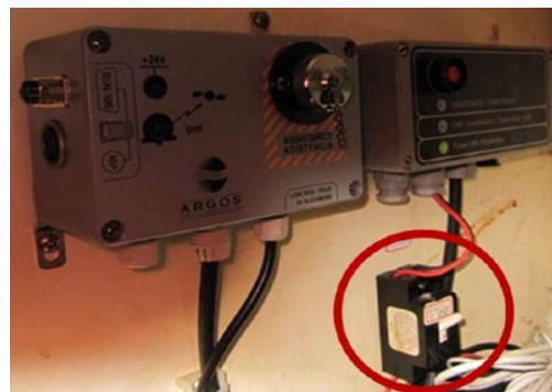
Figure 32 – VMS junction box with an on/off switch
